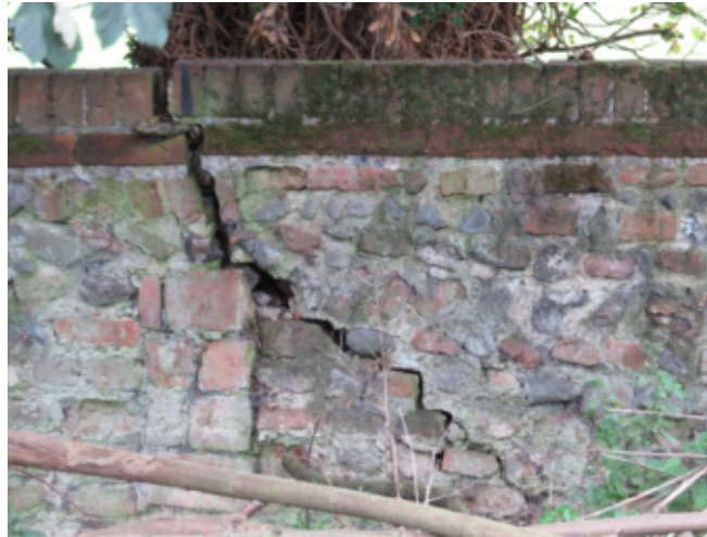
Cracked boundary wall due to tree growth
