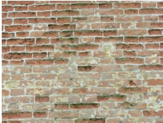
Brick delamination
