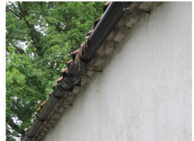
Broken gutters cause water to soak the walls, which leads to deterioration of the fabric
