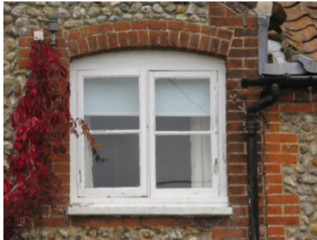
Example of external timber joinery requiring repainting
