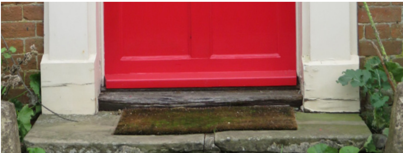
Rotting base to doorcase
