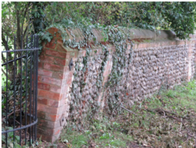
Leaning boundary wall
