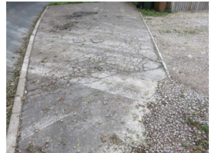
Poor surfacing to a large access splay
