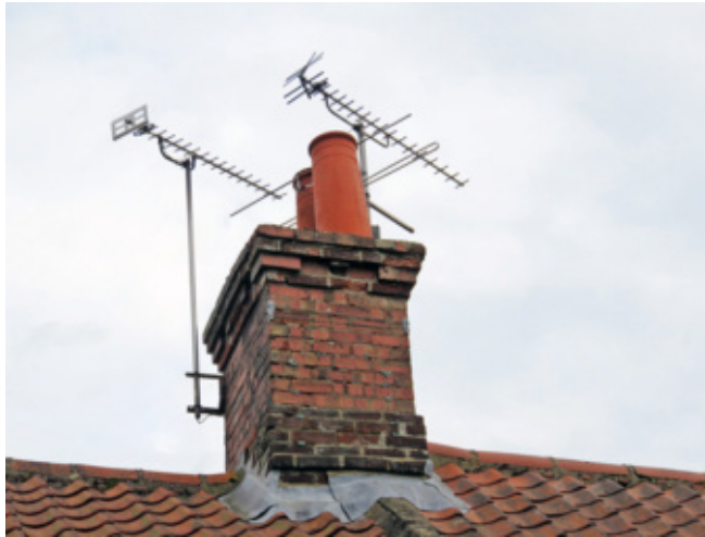
Television aerials and associated supports and cabling detract from the appearance of historic buildings and can cause damage to the historic fabric.
