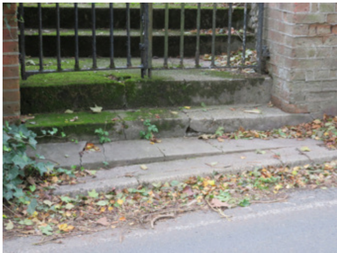
Cracking cementitious screed to steps
