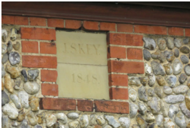
Late-nineteenth century date stone on the Key Buildings
