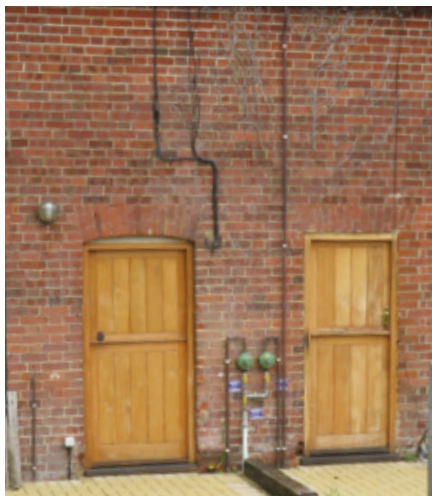
Prominent cables and inappropriate light fittings
