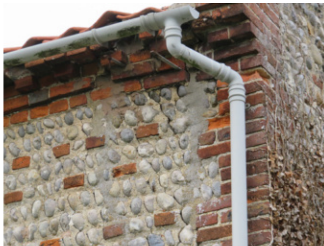
Cracks and cementitious repairs to a building
