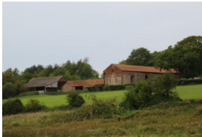
Barn range and farm buildings west of Thornage Hall
