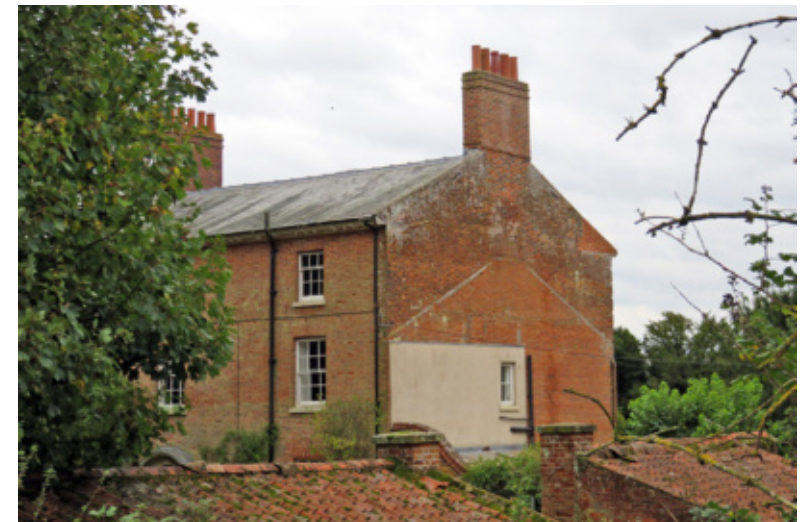
Rear elevation of The Old Rectory
