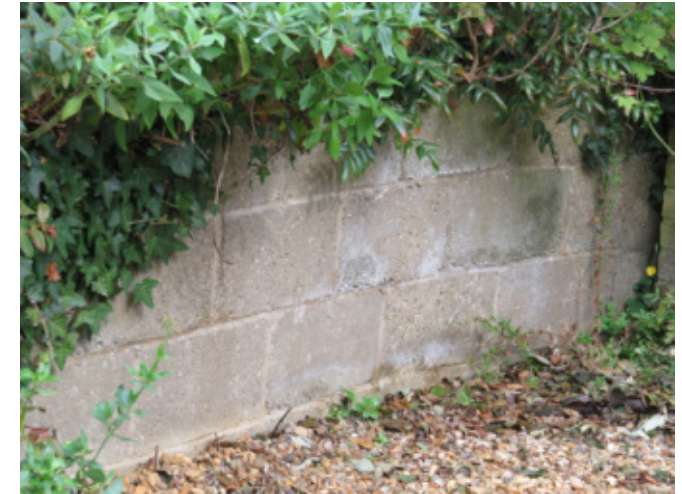
Example of a breezeblock wall
